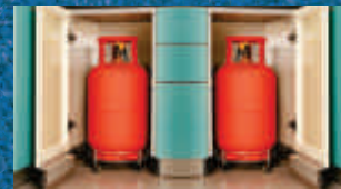
GAS CYLINDER OUTSIDE FROM KITCHEN ENSURE SAFETY
