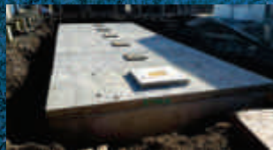
1.5 LAKH LTR. UNDERGROUND WATER TANK
